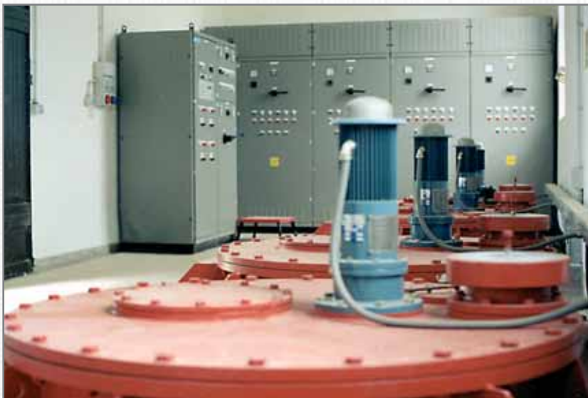
water-scooping station ↑ and switchboard
