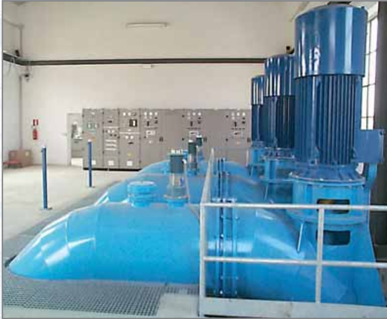
↑ pumping plant and control board in the background
