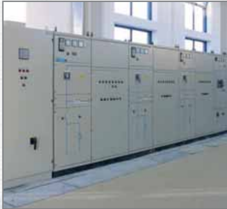
↑ low-voltage switchboard
