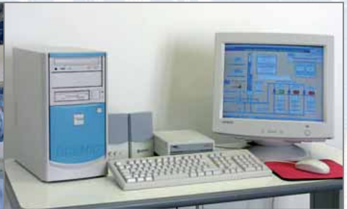
↑ PC plant control unit
