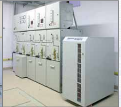
↑ medium-voltage switchboard
