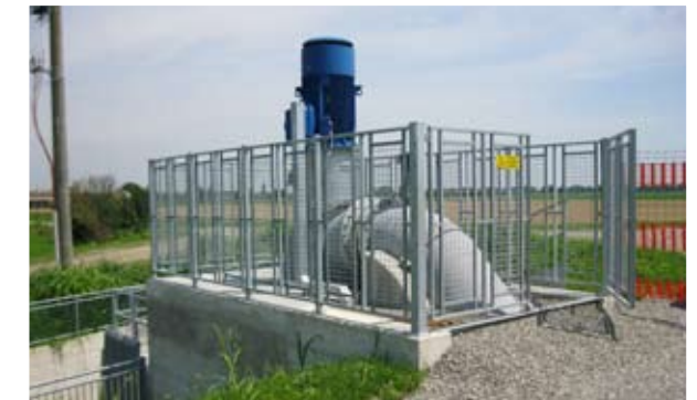
Consorzio della Bonifica Parmense Cantonale pumping station Amount of work € 204.207
