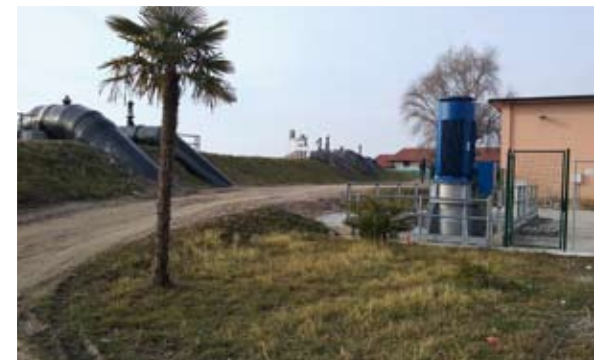
Consorzio di Bonifica Pianura Friulana Vittoria and Colomba pumping stations Amount of work € 798.401
