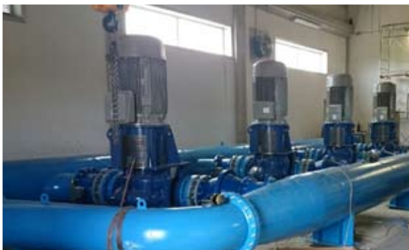
Extraordinary Commissioner for the realization of Basento-Bradano water works Pumping stations of 900 l/s and 1600 l/s Amount of work € 1.793.000
