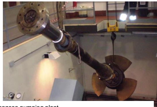
Repair of electric-pump Pellizzari type FIER 10.000 - Crevenzosa pumping plant
