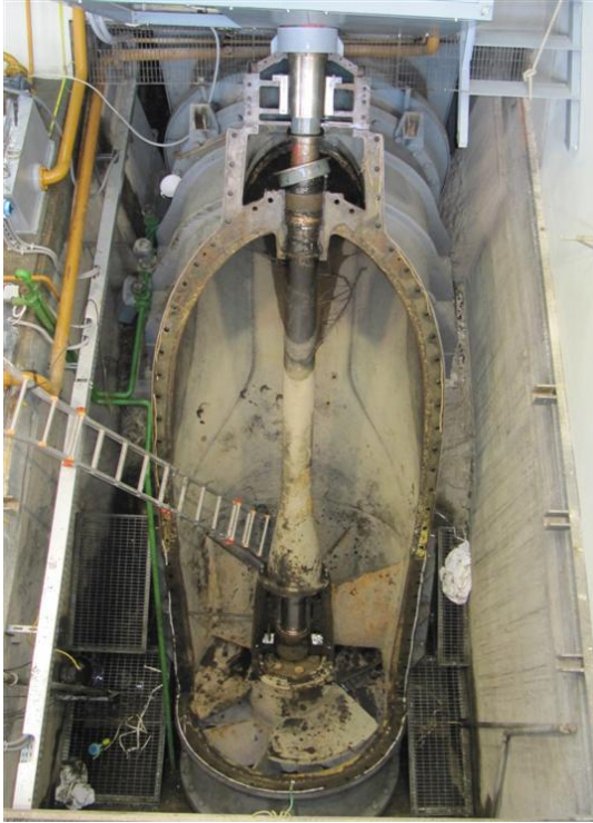
Repair of electric-pump Pellizzari type FIER 10.000 - Crevenzosa pumping plant
