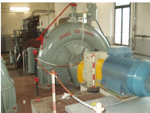
Various repairing and addition of new electric motor on old pumps.
