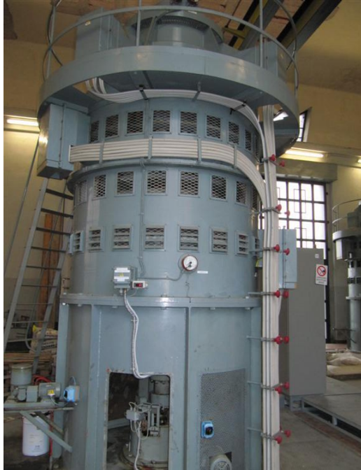
← Motor Pellizzari GAS 5000/22 n=267 rpm CV=1100 V=550
