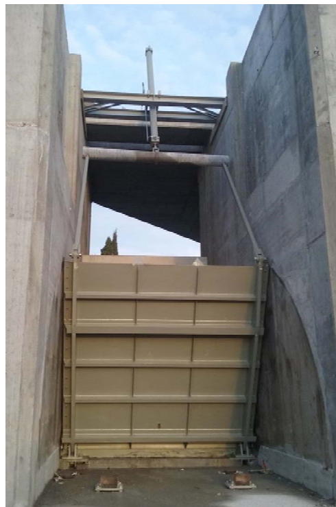
No. 1 Sluice gate for clean the river basin from stone and sand 2,77 x 3,30 m, in carbon steel S355JR, hydraulic control
