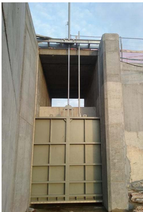
No. 1 Sluice gate for clean the river basin from stone and sand 2,77 x 3,30 m, in carbon steel S355JR, hydraulic control
