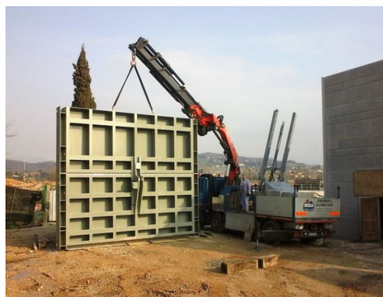
No. 1 Sluice gate for turbine protection 5,8 x 5,3 m, in carbon steel S355JR, hydraulic control
